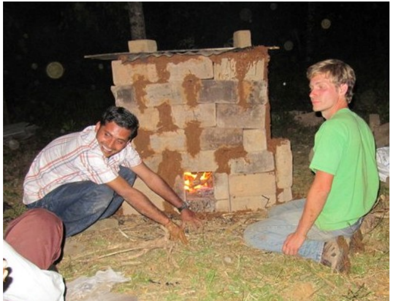
Fig 35: Heat retention structure made up of concrete brick built around the drum
