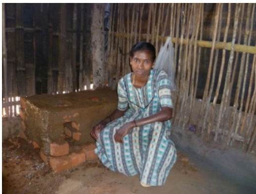
Fig 20: Stoves installed at 2 household in Srimadurai Area
